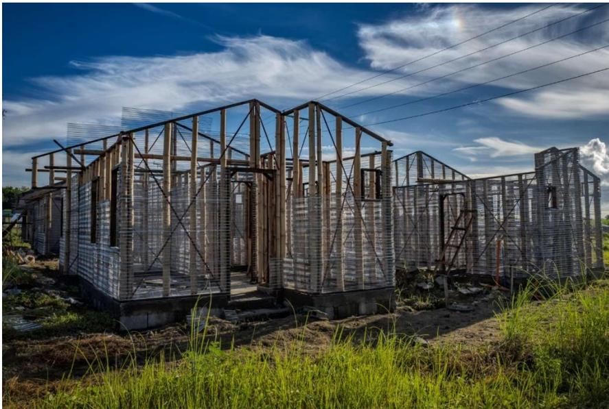
**Fig. 2.** Cement-bamboo frame technology (CBFT), Negros Occidental.
