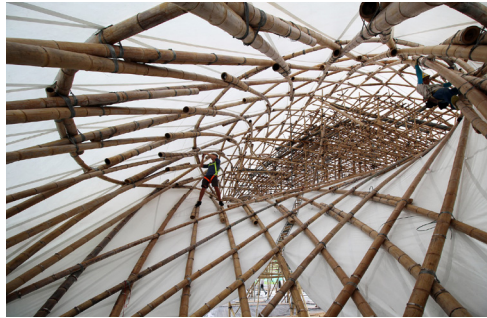
ZCB Bamboo Pavilion
