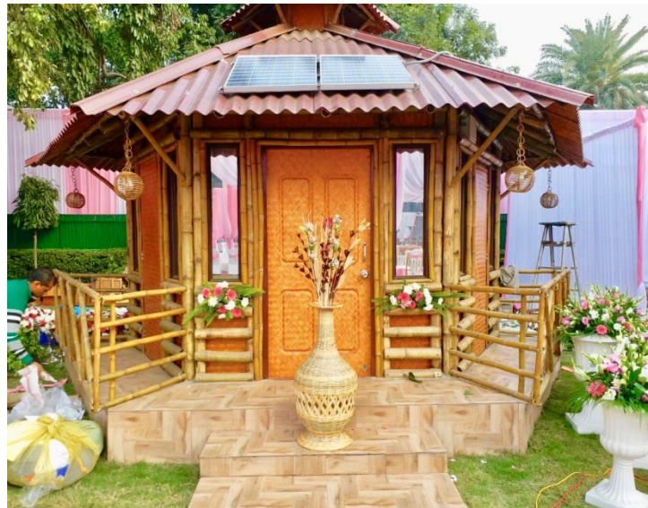
Prefab Bamboo Solar Hut, Delhi
