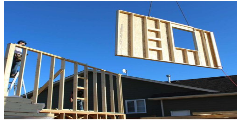
Level 2 - Panelized wall panel
