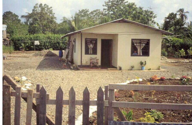
Plate 7: Undamaged Bahareque house after the 1991 Costa Rica earthquake (Gutierrez, 2004[5])
