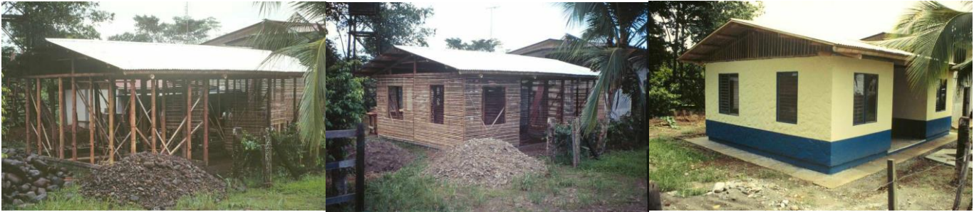
(a) Bamboo structure
