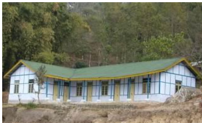
Plate 1: Ikra type housing (school building at Nandok, East Sikkim)(Kaushik et.al. 2006[2])
