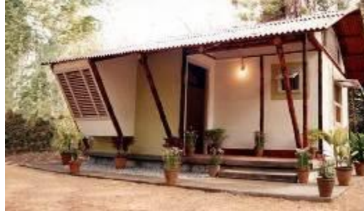
Plate 12: Demonstration house built by using IPIRTI-TRADA technology at IPIRTI, Bangalore; source: author
