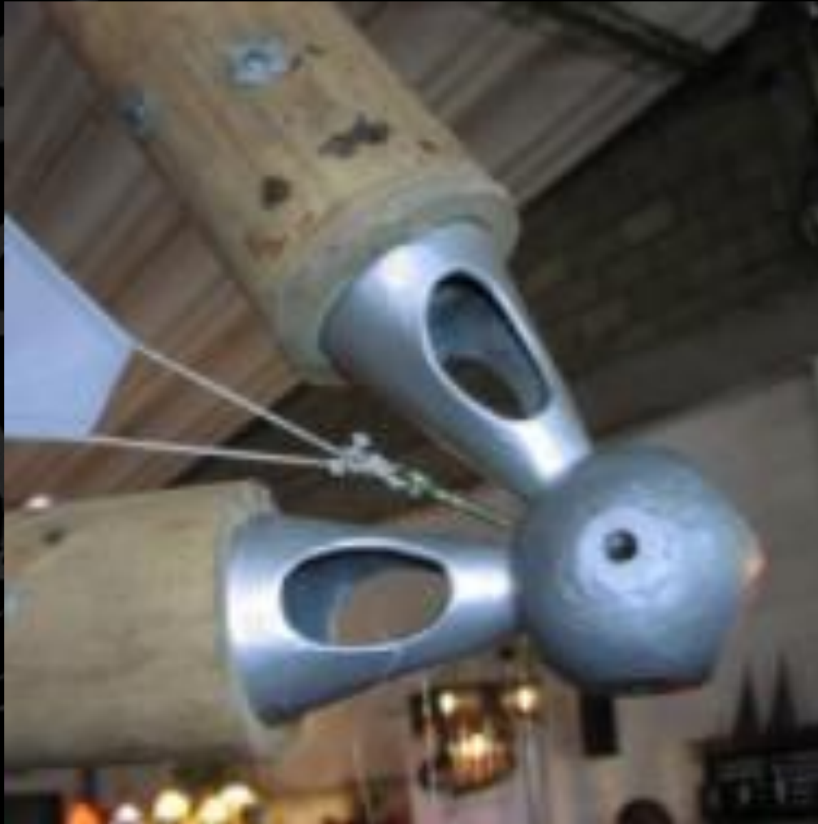
bamboo joint for space truss
